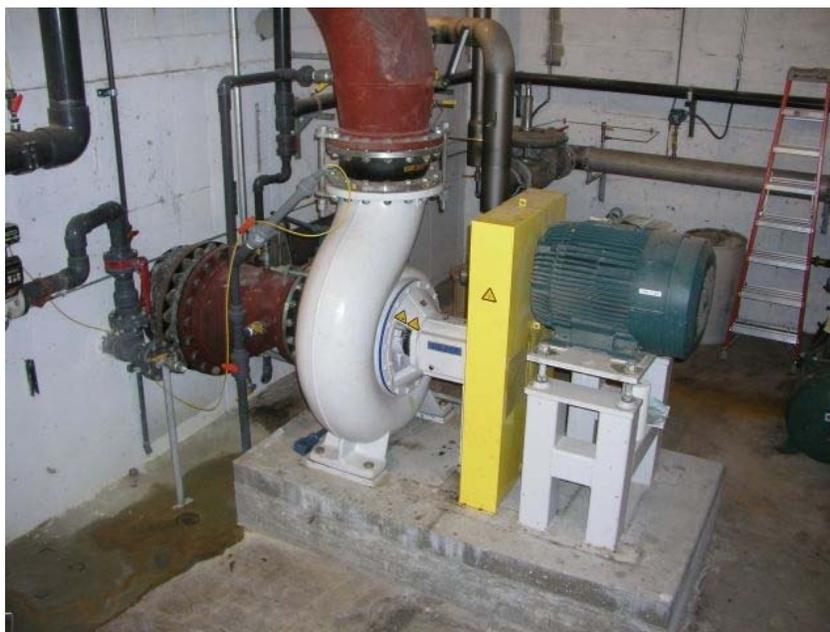
Figure 23 - Mixing pump for digester. Photo courtesy of Saputo Cheese USA, Inc.
