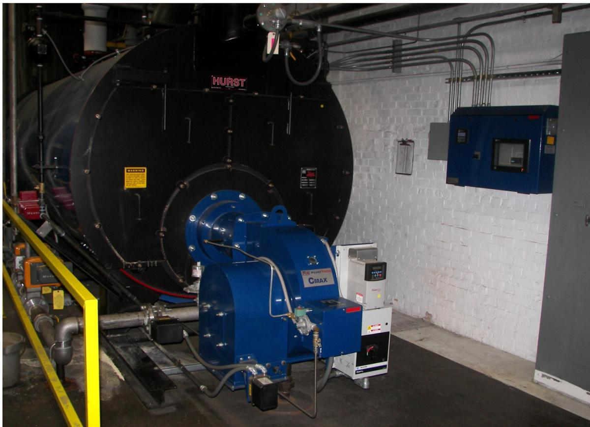
Figure 26 - Biogas hot water boiler. Photo courtesy of Seneca Foods.
