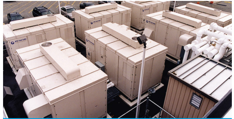
CHP fuel cell installation at Verizon data center. 1 Photo courtesy of Verizon Communications.
