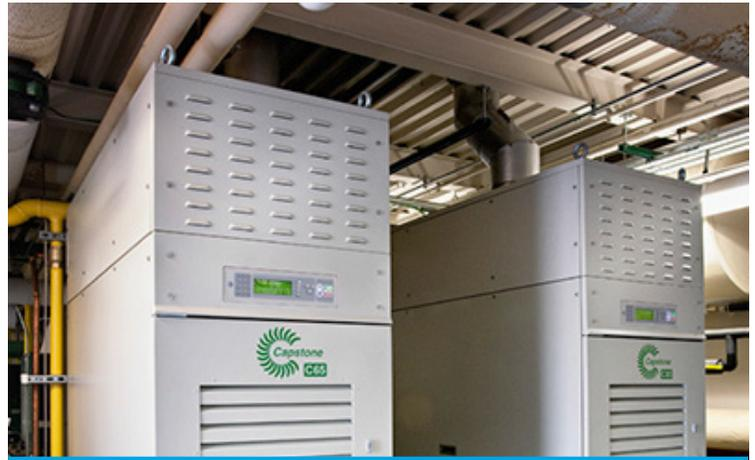
Microturbine CHP installation at a commercial facility.
