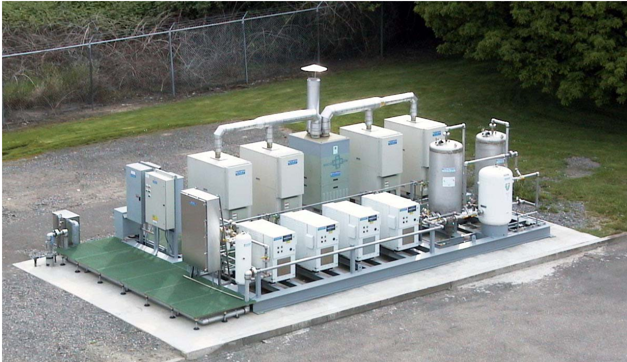
4 Capstone 30 kW Microturbines with Central Heat Recovery
