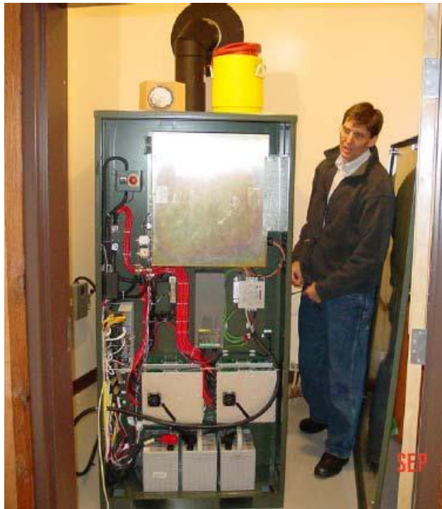
Initial Fuel Cell Installation
