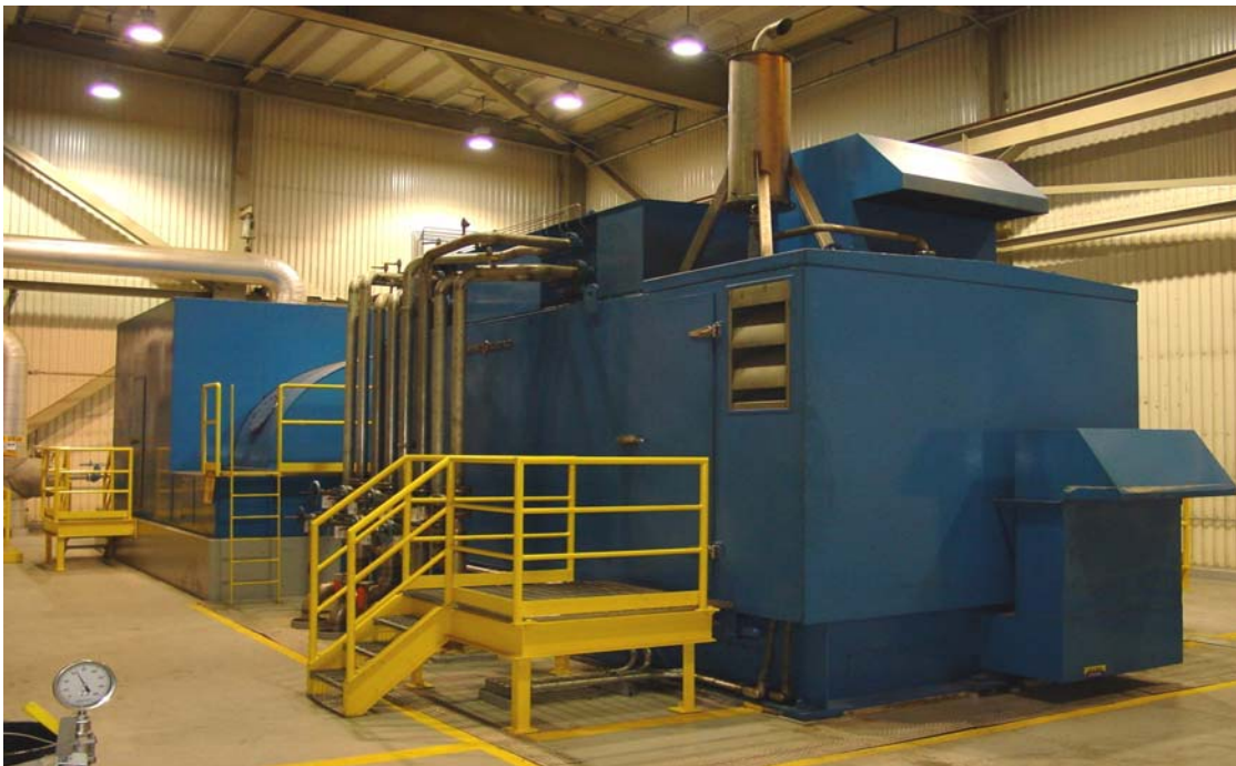
General Electric Steam Turbine Generator
