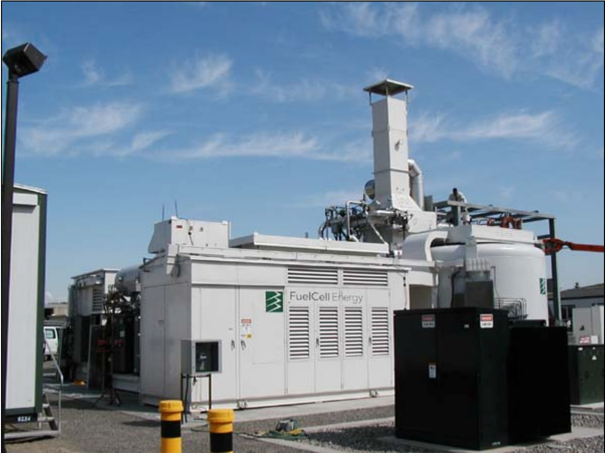
This King County photo shows the electrical balance of plant.
