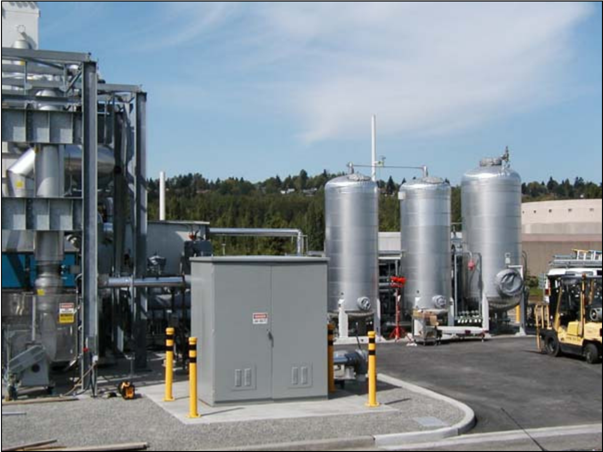
This King County photo shows the sulfa-treat vessels (for digester gas scrubbing).
