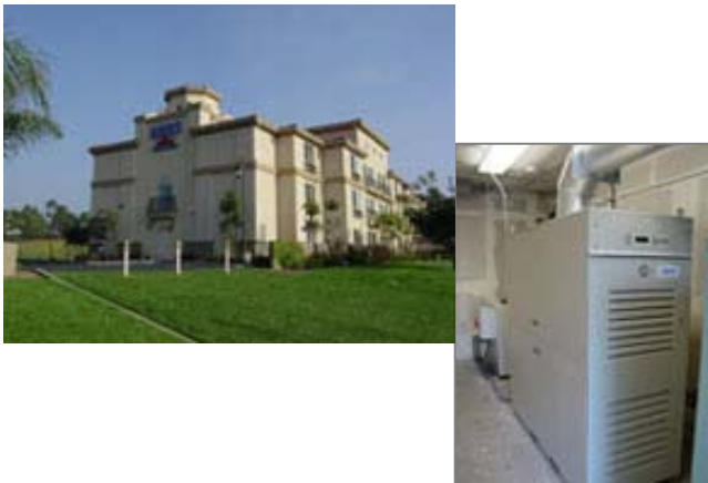
Figure 6. –C60 CHP System at Inns of America
